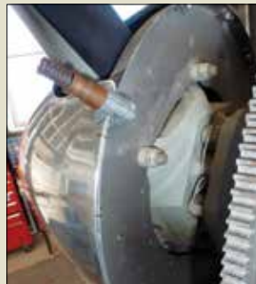
Cleco clamps were used to hold the dome in place while marking locations for the screw holes.
